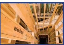
wind resistance, strength, and appearance in tall walls, and eliminates the "hinge" created by platform framing. Versa-Stud wall framing offers 182% more bending strength and 112% more stiffness than no. 2 SPF 2x6 studs. Versa-Stud
